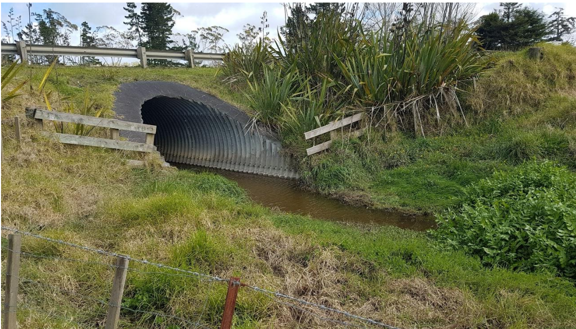
Figure 3.3: Culvert underneath existing Pine Valley Road
